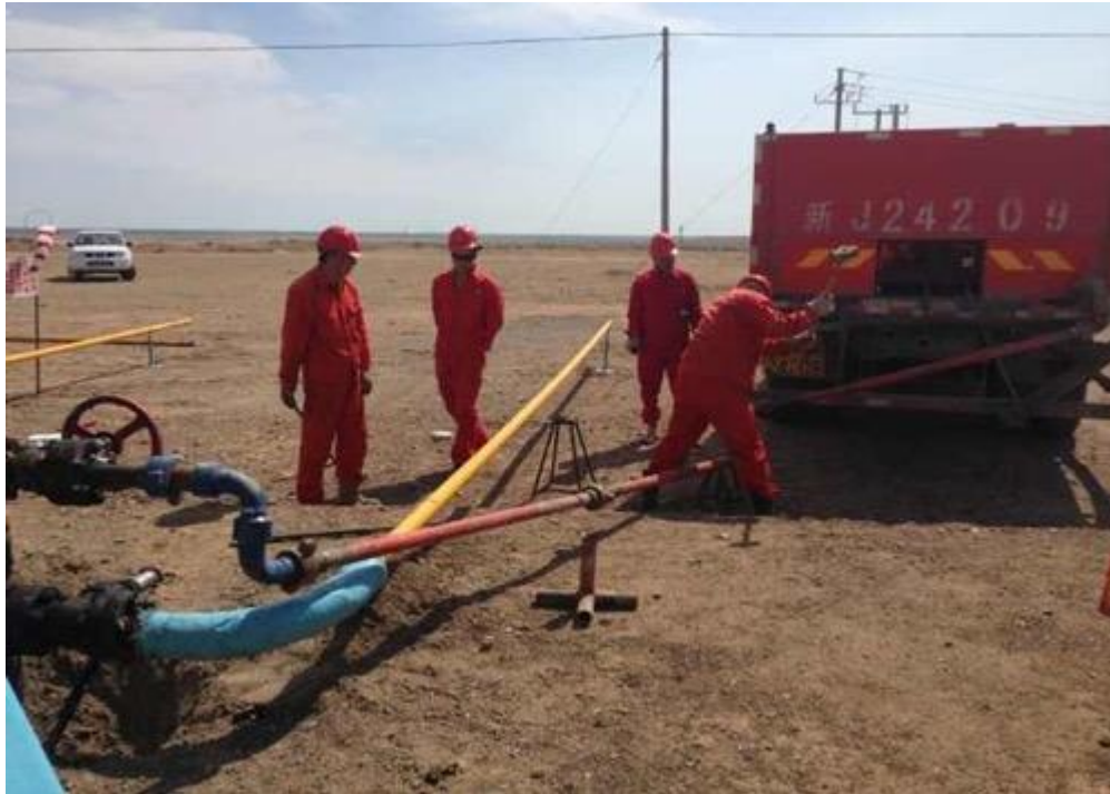
Slug process physical pipeline connection diagram
